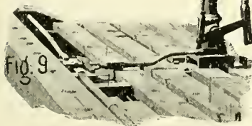
BLACK'S AUTOMATIC MECHANICAL SIGNAL AT "DANGER."
